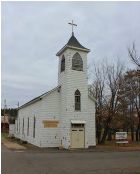
Michigamme Library - An example of an adaptive reuse for a public building
